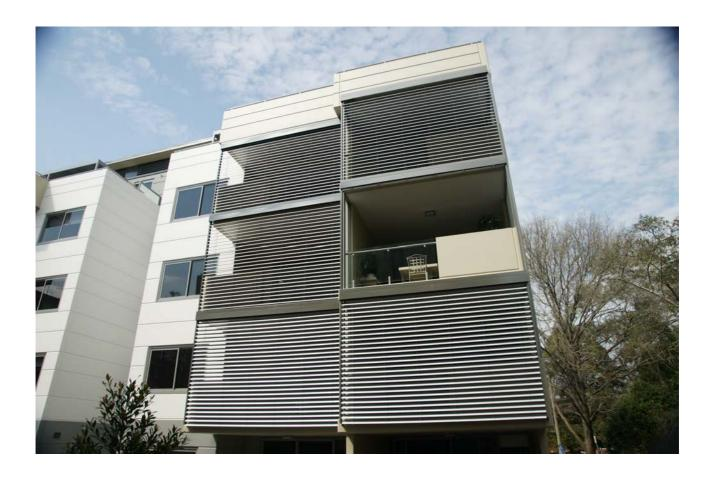
2/ The world renowned Hagofix® slat support system of spigot tape with stainless steel connector has been modified and designed by SURE SHADE® . The size , metal properties and design of the stainless steel connector has been developed by SURE SHADE® to increase the wind load capacity of the system and the distance between spigots has been increased to 107mm to suit rotation of the larger slat.
