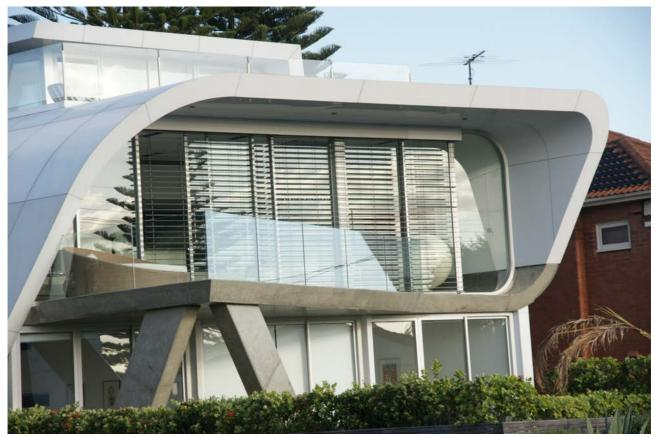
The blind slat profile **SURE SHADE® Basic 100F** is 100mm wide and can only be controlled by ladder braid and is manufactured from a special aluminium alloy which provides the slat with flexibility of movement under wind load or use. The advantages of the flexible slat is that the slat is able to absorb impact by deflecting and rebound back to the original convex shape.
